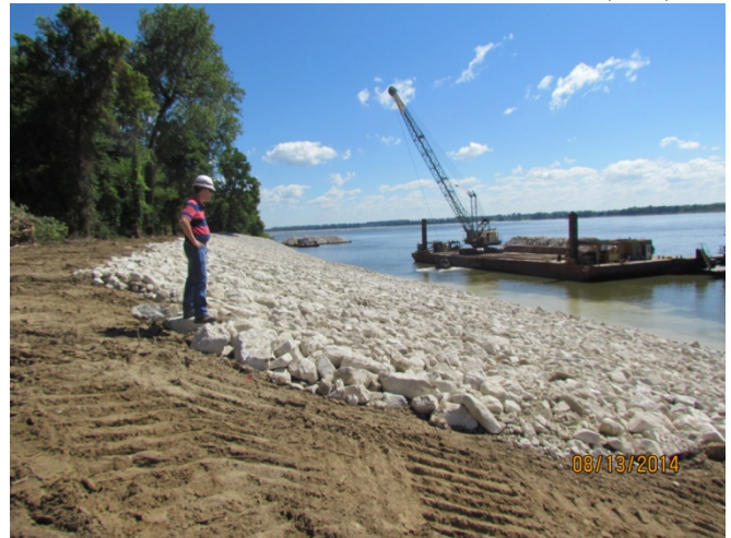
Island 18, MO Stone Revetment Construction
